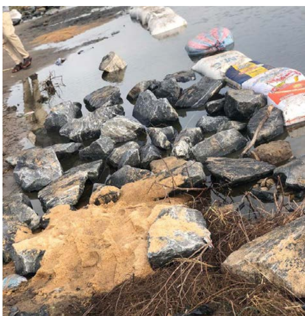
Use of sandbags and stones for pavement
